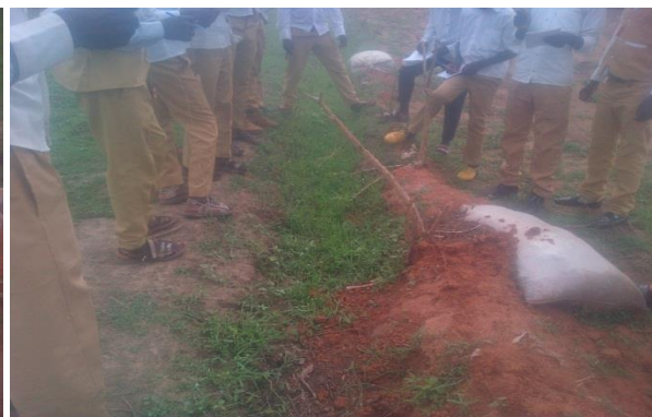
Fig 6: Shows the adoption of sand bags techniques on controlling soil erosion
