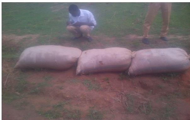
Fig 6: Shows the adoption of sand bags techniques on controlling soil erosion
